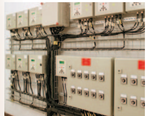
Monitoring and control capabilities up to 130 circuits per control unit
